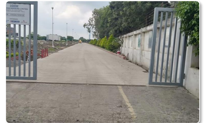
New Concrete Road At Entrance
