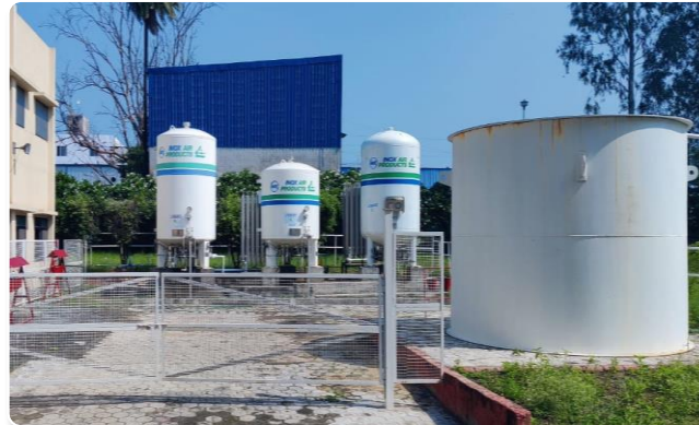
Expansion of Oxygen Tank
