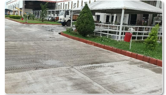
New Concrete Road inside Plant
