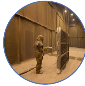
Shot blasting of carbon steel up to 5000 x 4000 x 2000mm
