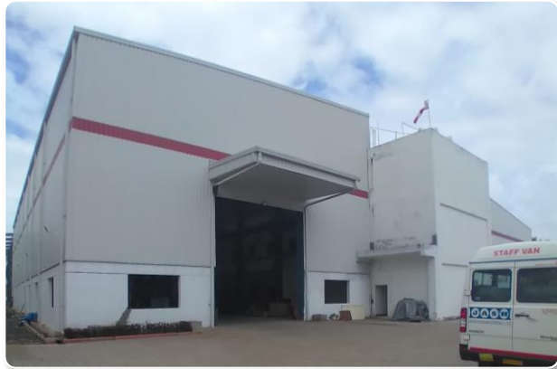
Plant Expansion for Cast Iron Products
