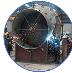
Fabricating capacity for jobs up to 50 tonnes weight
