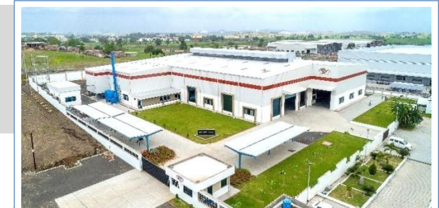
UNIT-4 Rodney Hunt Plant BUILT UP AREA: 50,000 Sq. ft. Turnover Capability : ₹ 100 Crore
