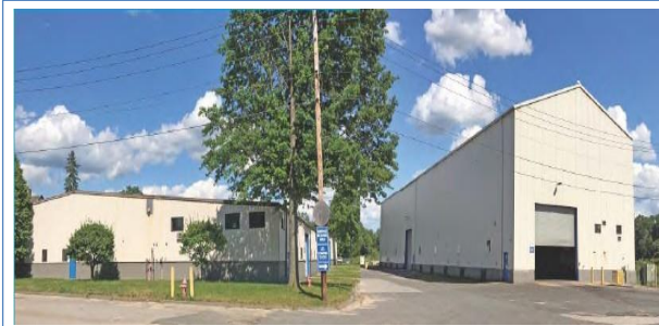
Rodney Hunt Plant, Orange, MA USA BUILT UP AREA: 60,000 Sq. ft. Turnover Capability : USD 10 Million
