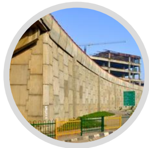
Reinforced Earth Walls
