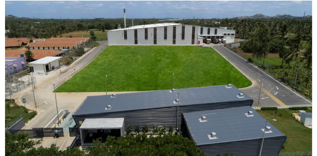
Unit III - Hosur facility - Soolagiri plant
