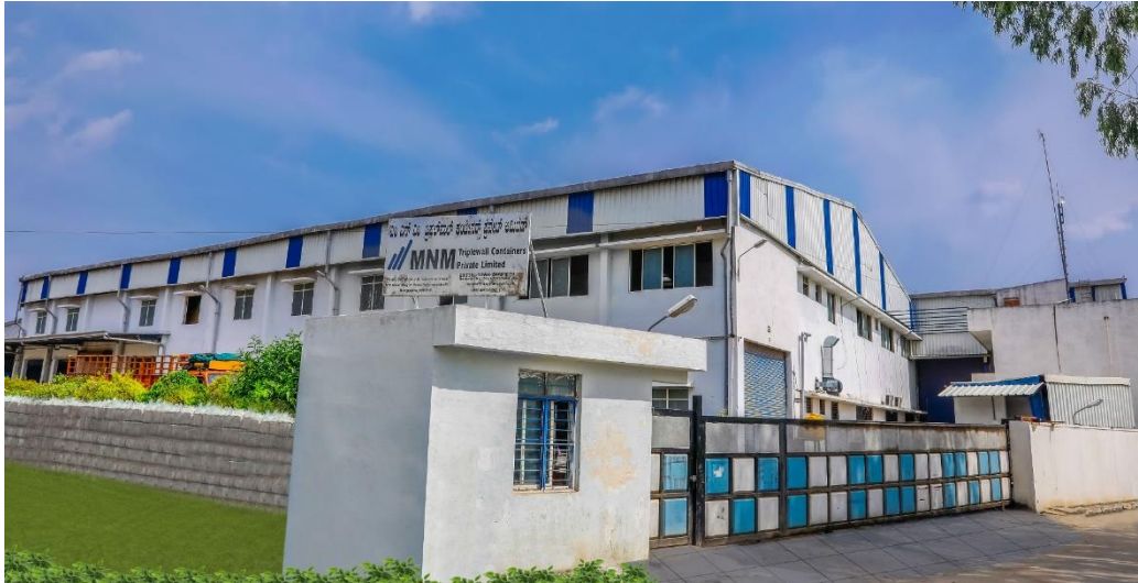
Unit I - Bangalore facility - Attibele plant
