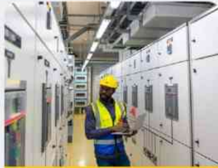
TURNKEY E&I PROJECTS
