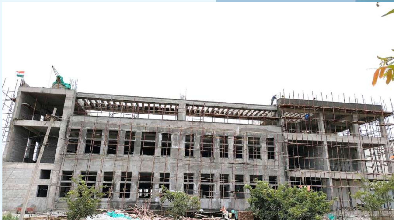
Construction progress at the proposed integrated facility
