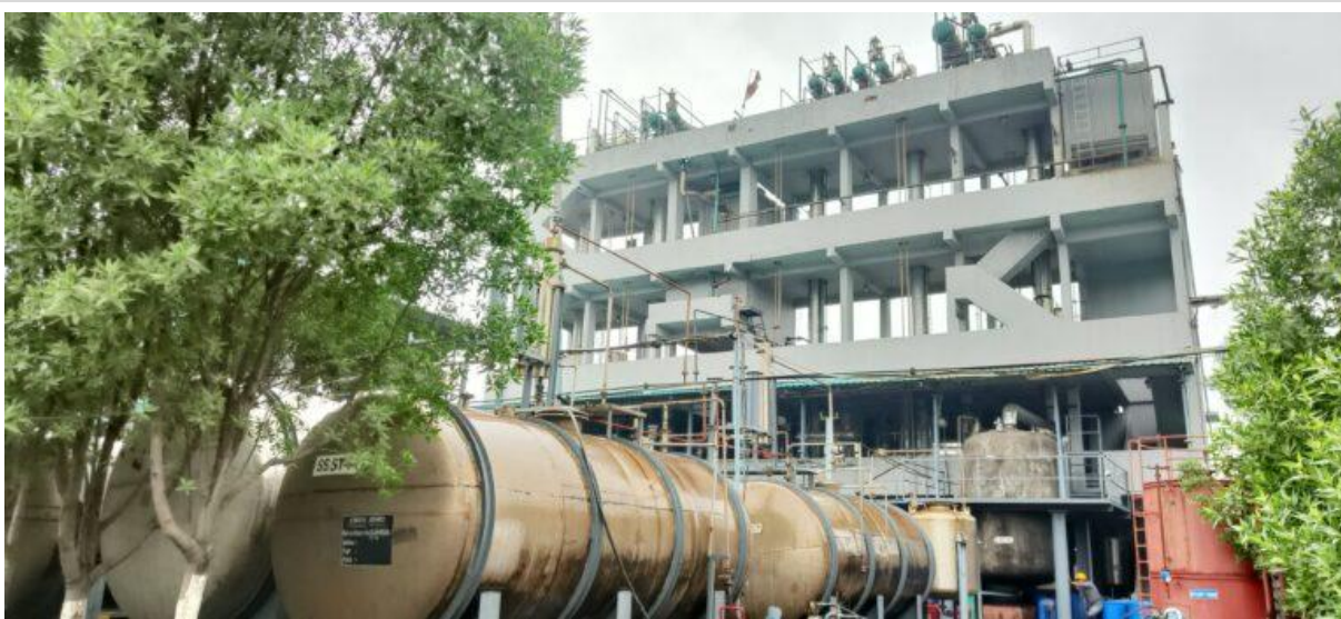
Multi-stage fractionating distillation and reactor unit used in the solvent recovery process.
