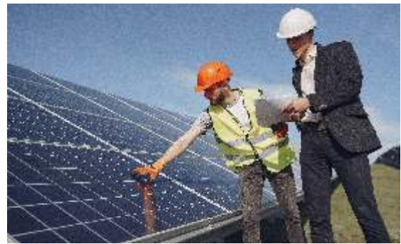
Concept to commissioning Solar Plants
