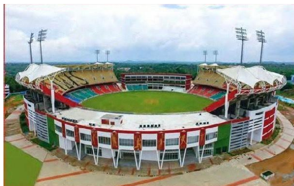
Architectural and fabricated structures
