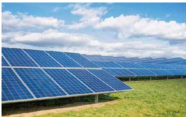
Solar and infrastructure structures
