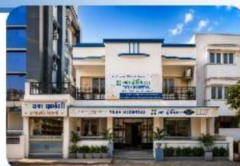
YASH HOSPITAL PADRA , DIST : VADODARA
