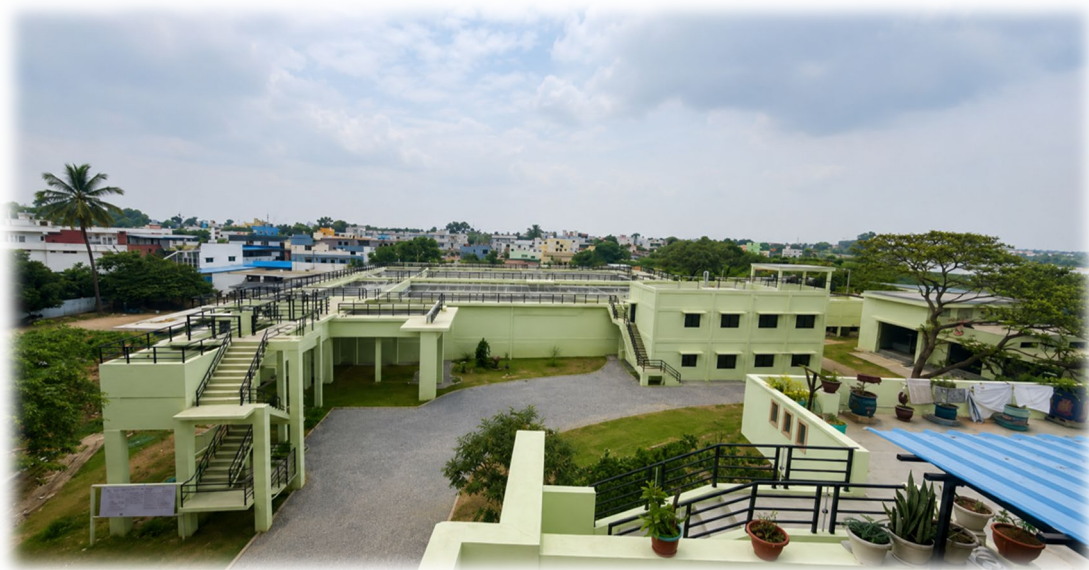
Design, Engineering, Construction, Operation & Commissioning of 32.6 MLD SBR-Based Sewage Treatment Plants (12.5 MLD & 20.1 MLD) Package III – Hosur City Municipal Corporation Location: (📍) Hosur, Tamil Nadu
