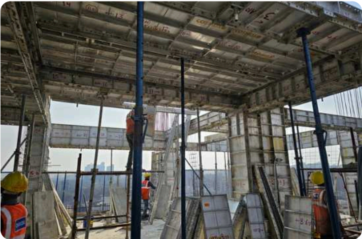
Equipment name : Aluminum Monolithic Formwork Country of origin : Malaysia Amount invested : ₹7.6 crores
