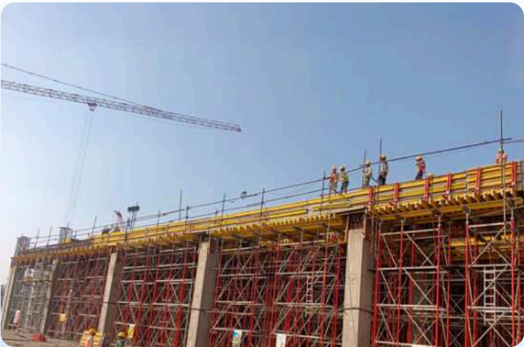
Equipment name : Peri Up MI System for Beam Bottom Country of origin : Germany Amount invested : ₹6.7crores
