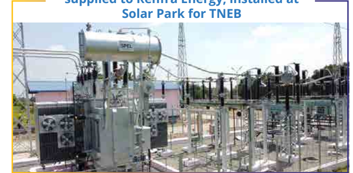
10 MVA 110/33-11 kV Power Transformer installed at Malarbettu, Ooty for TNEB
