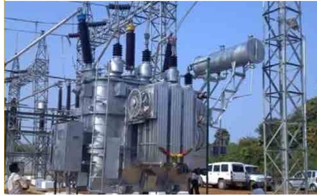
40/50 MVA 110/33 kV Power Transformer supplied to Velan Infra, installed at Solar Park for TNEB
