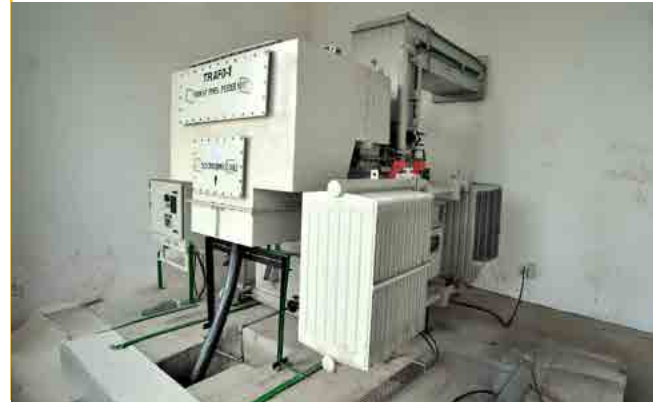
1500kva 33/0.433kv Transformer Supplied To Siemens (Spain Based Company)
