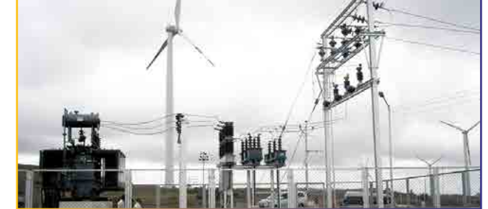
950kva 33/0.69kv - Windmill Transformer Supplied To Gamesa (Spain Based Company)
