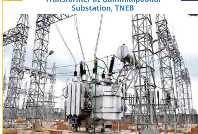
40/50 MVA 110/33 kV Power Transformer supplied to Velan Infra, installed at Solar Park for TNEB
