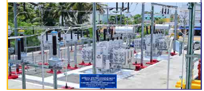
950kva 33/0.69kv - Windmill Transformer Supplied To Gamesa (Spain Based Company)
