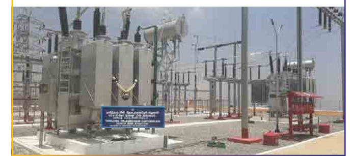
16 MVA 110/22-11 Kv Power Transformer Installed At Villarasampatty For TneB
