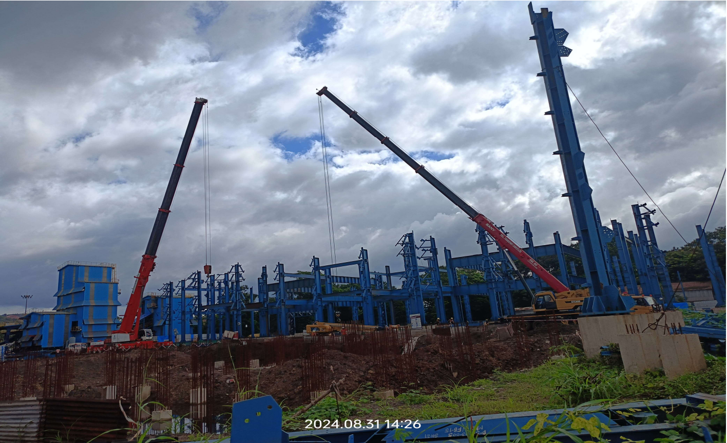
TSL Joda Furnace Building
