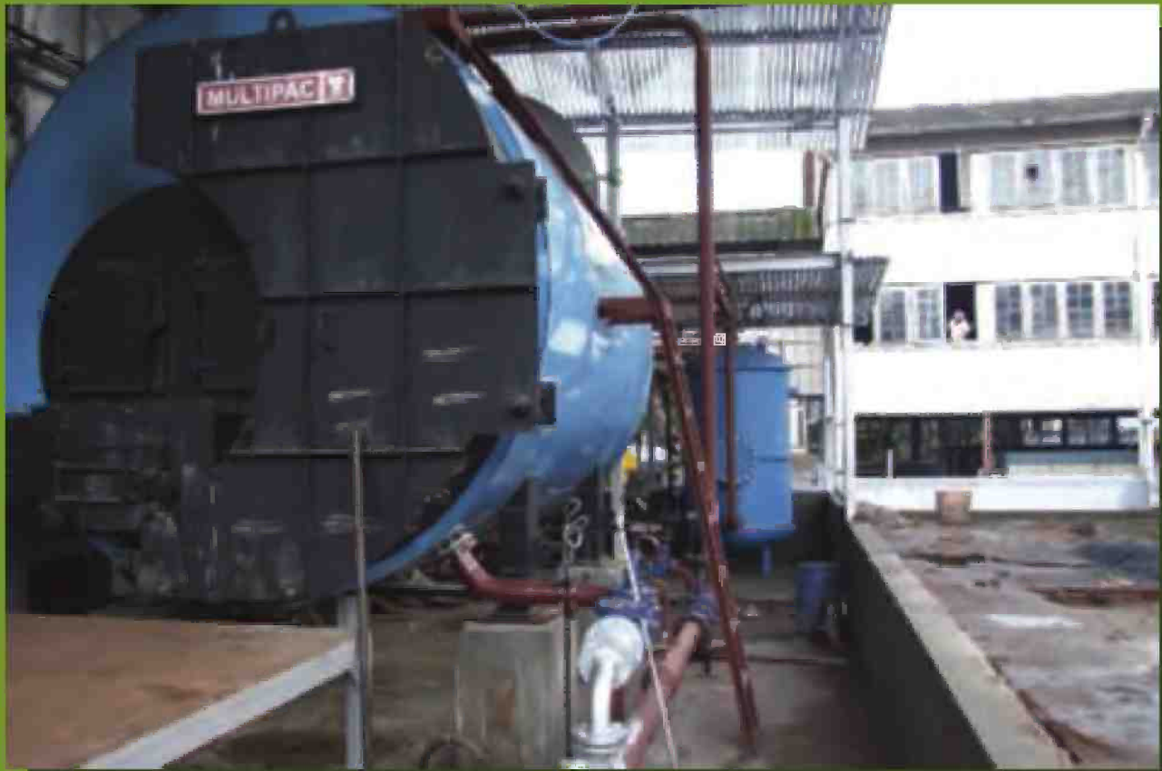
▲ Hot water boiler - Wallardie
