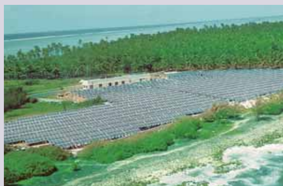
Country's Largest Diesel Grid-Interactive Solar Power Plant of 760 kWp capacity, commissioned by BHEL at Lakshadweep
