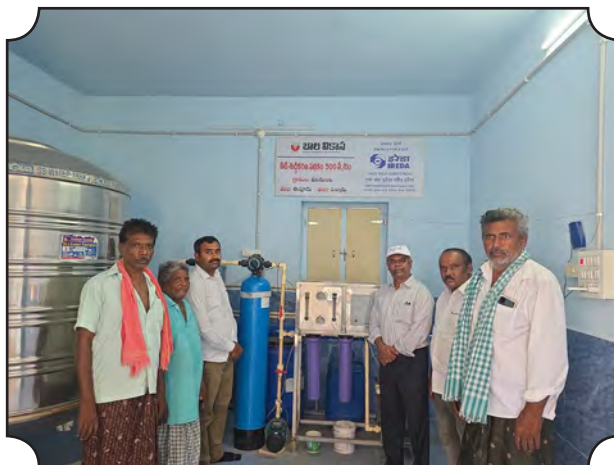
Installation of R.O. Water Treatment Plants in villages of Vinukonda Palnadu District, Andhra Pradesh
