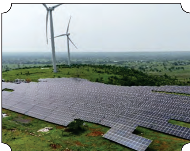
IREDA funded 2.3 MW Solar PM-KUSUM project in Shajapur, Madhya Pradesh
