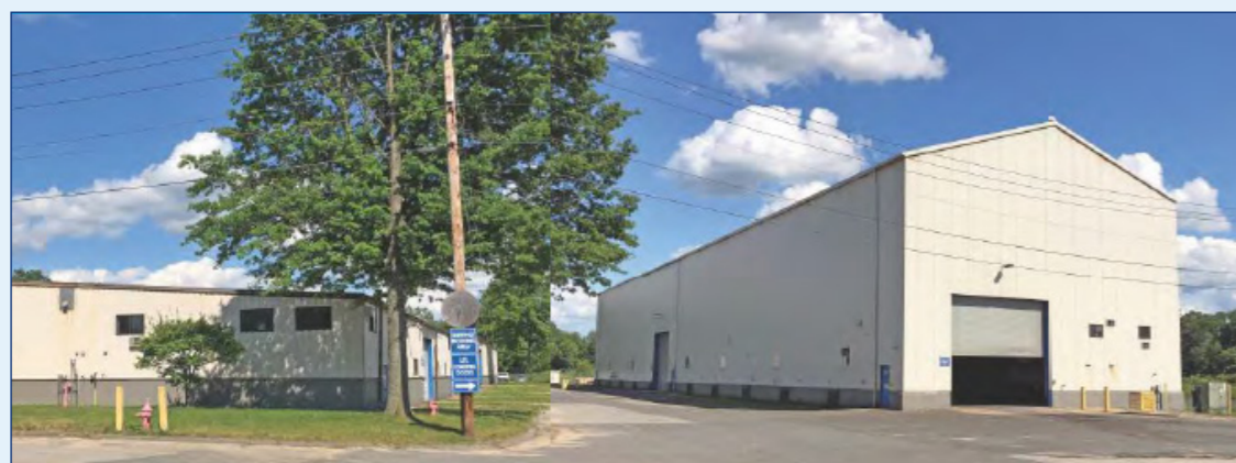
Rodney Hunt Plant, Orange, MA USA Built Up Area: 60,000 Sq. ft. | Turnover Capability: USD 15M (₹ 125 Crore)
