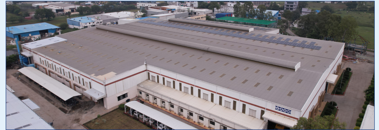
UNIT-2 FABRICATED PRODUCTS PLANT Built Up Area: 185,000 Sq. ft. | Turnover Capability: ₹ 350 Crore
