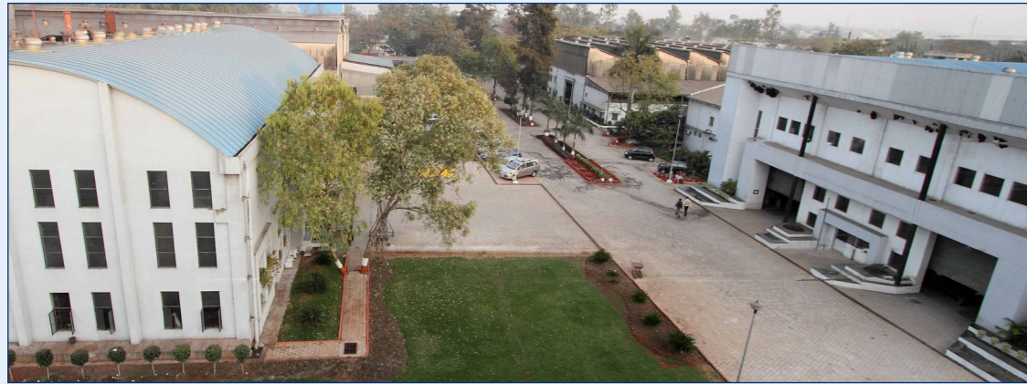
UNIT-1 CAST PRODUCTS PLANT Built Up Area: 125,000 Sq. ft. | Turnover Capability: ₹ 75 Crore
